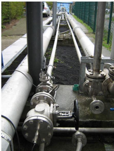
Fig. 13: Test valve at the end of the branch line [7]
