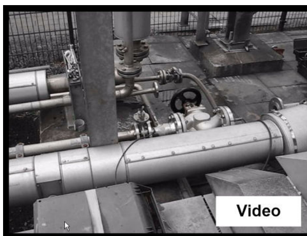
Fig. 13: Test valve at the end of the branch line [7]
