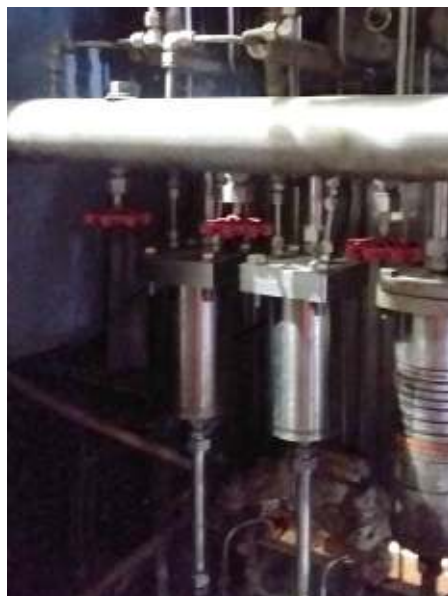
M4 Knick Coolers for sample conditioning
