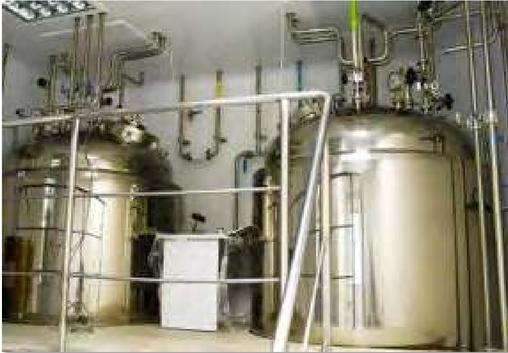
Figure 5: Pharmaceutical tanks installed in close quarters.
