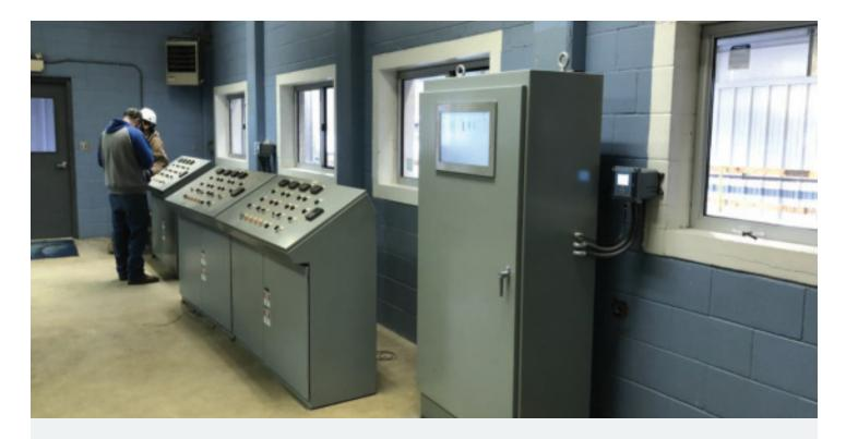
**Upsized features; downsized space.** The three older filter consoles shown to the left are being replaced by the single new filter controller, to the right. Touchscreens mounted on the new consoles use the same Ignition interface screens as those in the control room, streamlining implementation of system-wide control screen changes.
