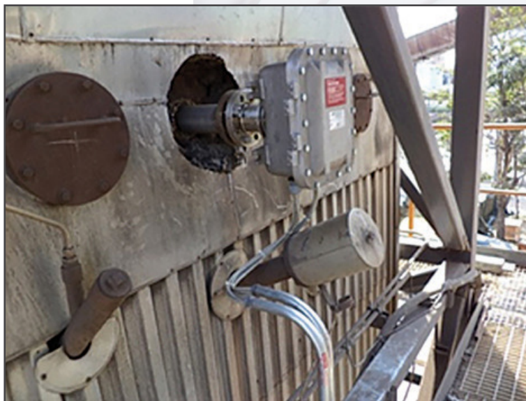
Flue gas monitoring at a cement plant
