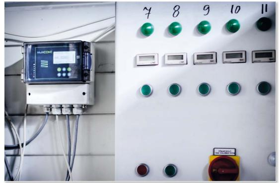
The raw materials are mostly arriving by tank trucks. So a "switch" been built into the NIVISION system which changes the silos colour signal to green if a whole truck of material can be loaded into it securely.
