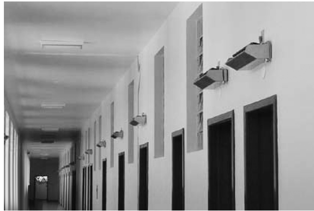
Fig. 8 Upper-Air UVC Devices in Naturally Ventilated Corridor of TB Facility in Brazil (Centers for Disease Control and Prevention)
