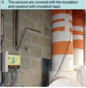
The complete installation takes ~4 hours. This includes wiring and programming the BTU meter. A feature of Flexim BTU metering is the ultra low flow velocities that the meter accurately picks up. The meter just installed shows velocities down to 0.023 ft/sec.
