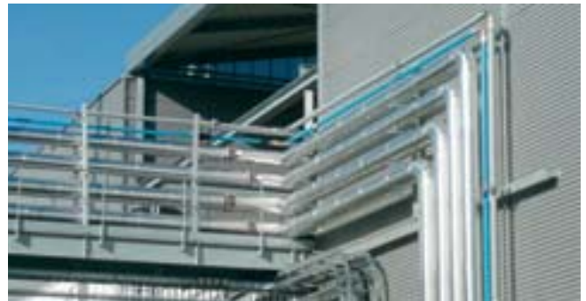
Outdoor installation Transair Ø 168
